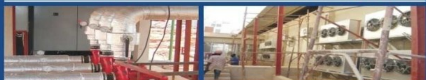
PRIMARY PUMP INSTALLATION AT NIGERIA JUDICIAL COUNCIL
