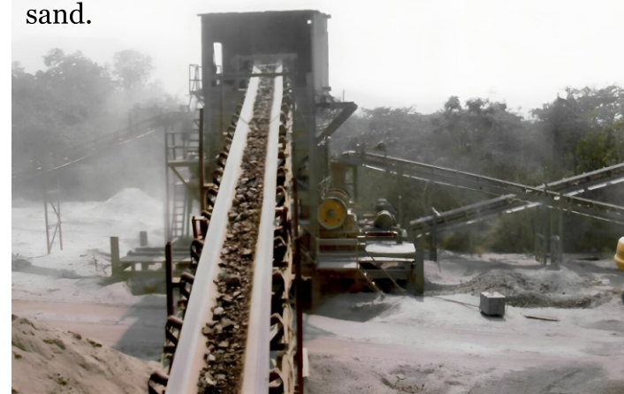
Conveyoe Belts & Crush Plant
